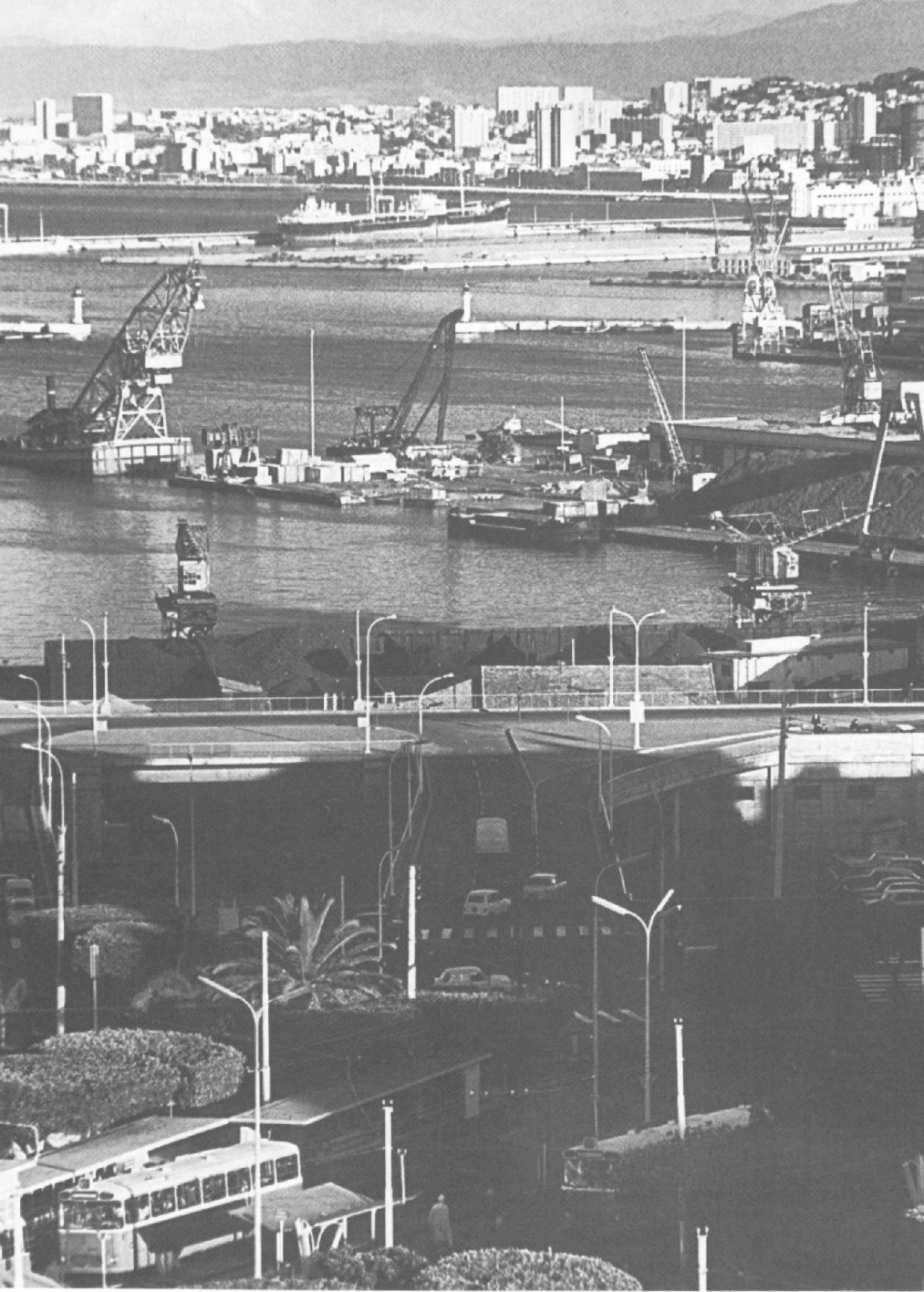
Port of Algiers, the country's principal maritime facility for general cargo and passengers Courtesy United Nations
